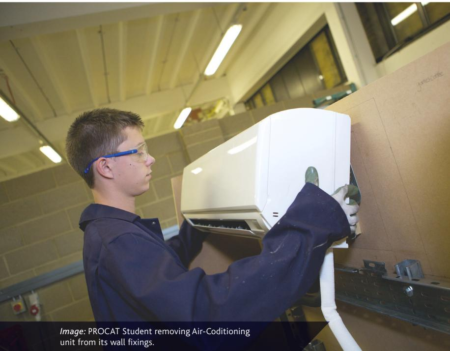
Image: PROCAT Student removing Air-Conditioning unit from its wall fixings.
